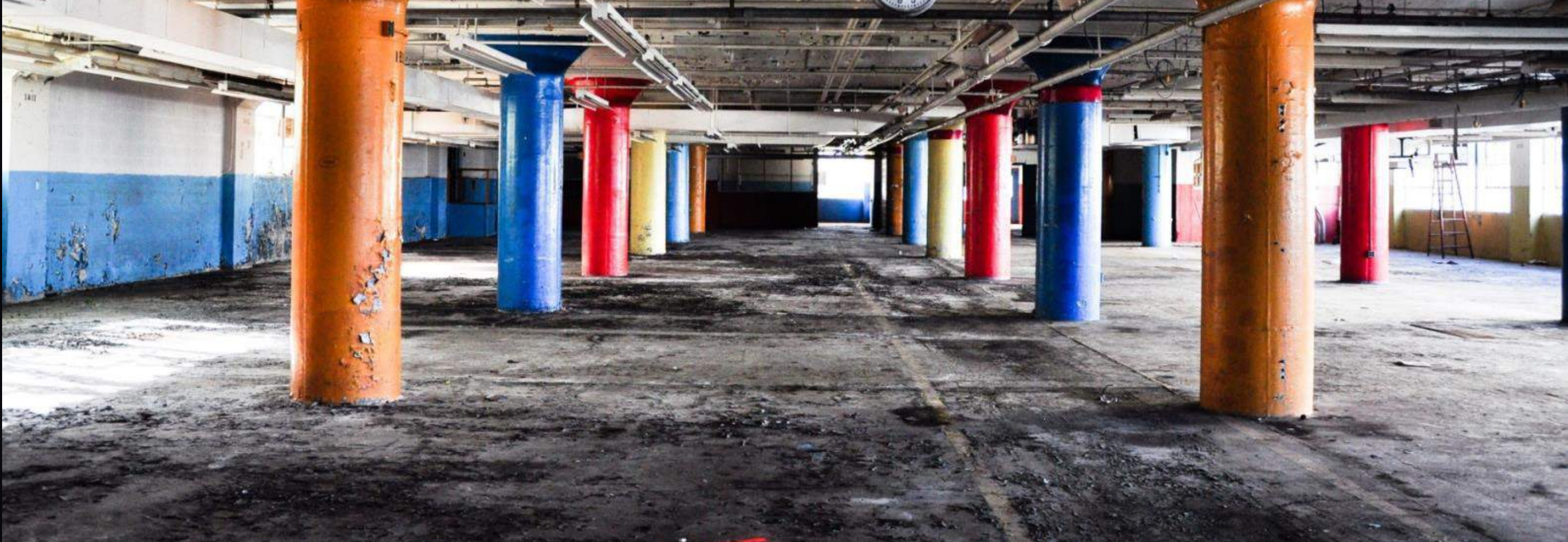
INTERIOR OF EXISTING STRUCTURE 11.18.2014
